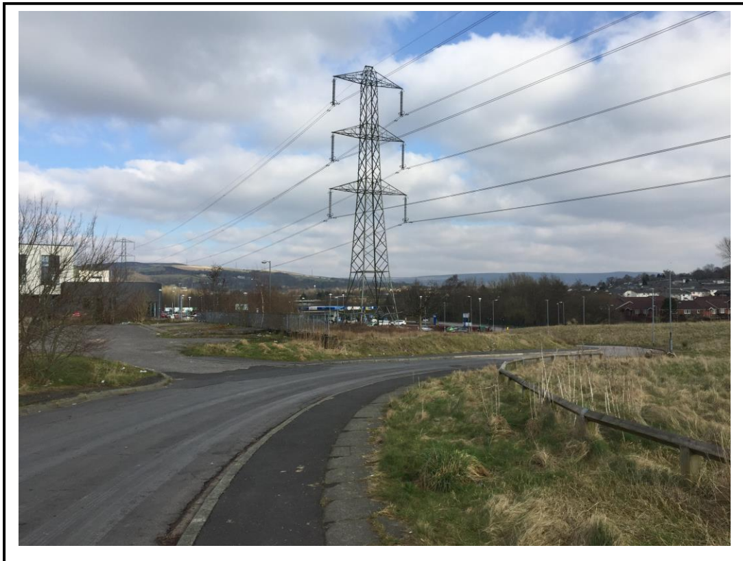
Photo 4 – view into the site from the southern end of Chain Bar Lane.
