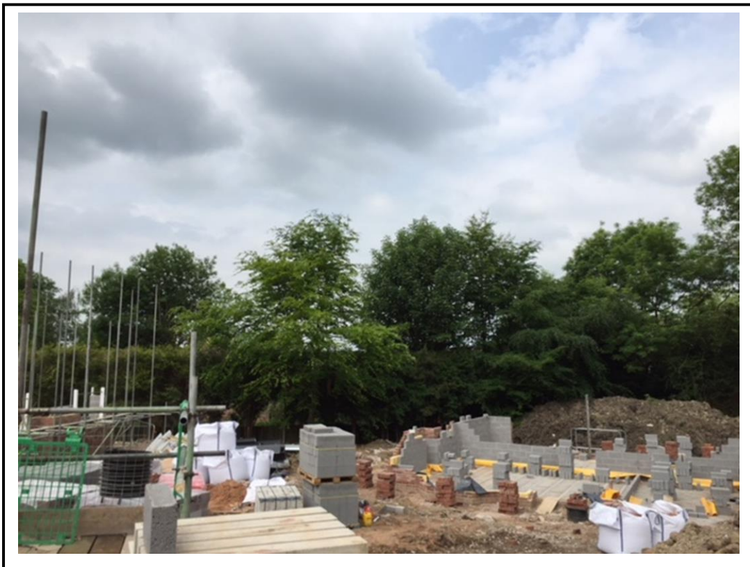
Photo 4 – view from within the site looking towards the north western boundary
