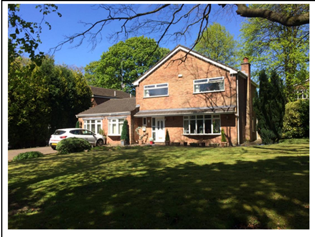
Photo 5 – existing property at no. 2 Ralphs Lane
